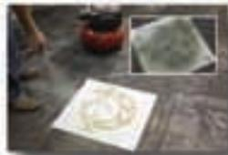
**Step 2:** Spray layers of SmartColor™ over the Modello in a faux, random pattern.
