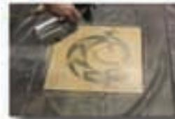
**Step 3:** Spray layers of SmartColor over the surface for a mottled, faux effect.
