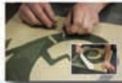
**Step 3:** Carefully peel the Modello pieces from the concrete using a pick tool.
