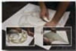
**Step 1:** Apply the "Modello" to smooth concrete—burnish with pressure for good adhesion.
